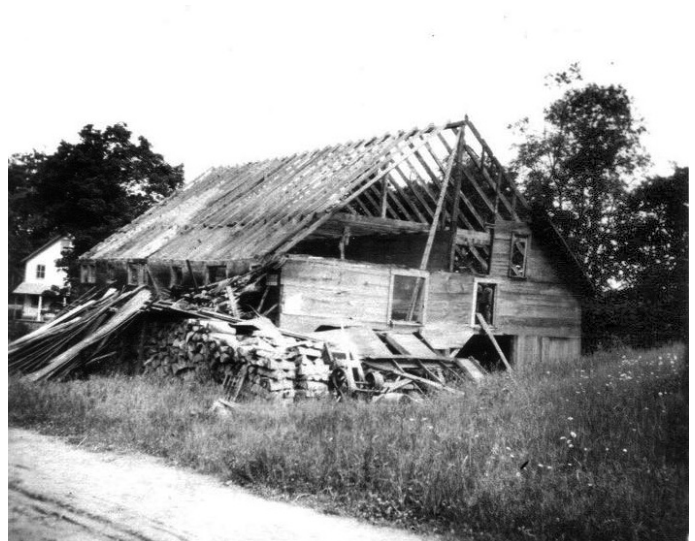
Messer mill demolition, ca. 1914.
