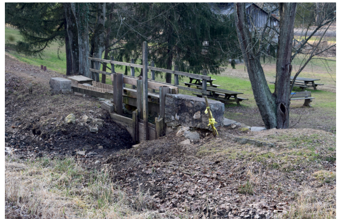
Spillway gate (millrace side) after being dewatered.
