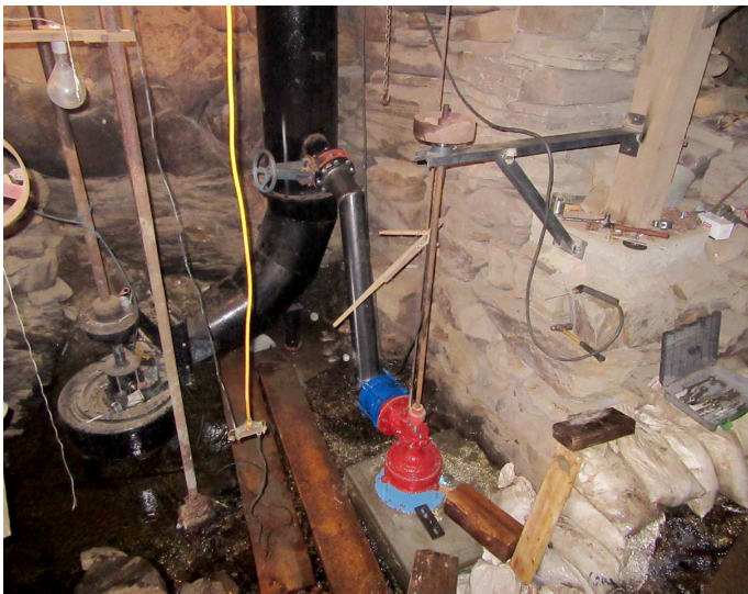
21-in. Wetmore turbine installed on left; 9-in. Tyler wheel on right.
