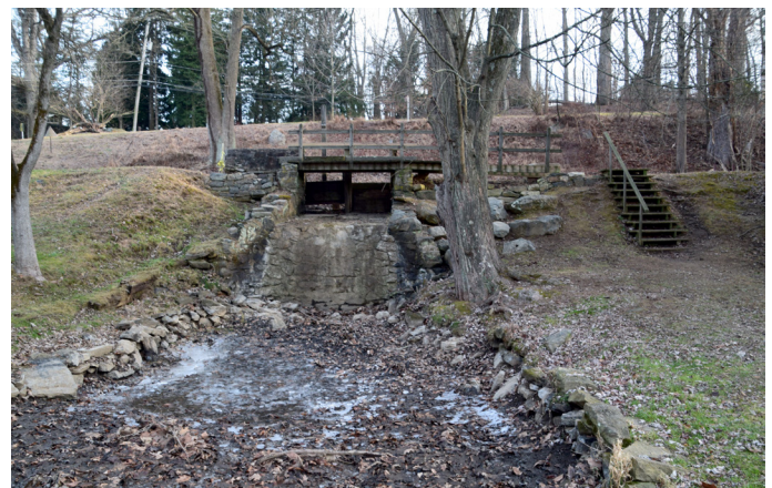
Spillway gate (downstream slope side) after being dewatered.
