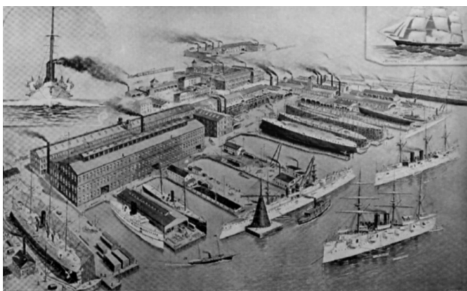
Yard of the William Cramp & Sons Ship & Engine Building Co., 1892. The conical object is Atlas, the floating derrick (built 1892).
