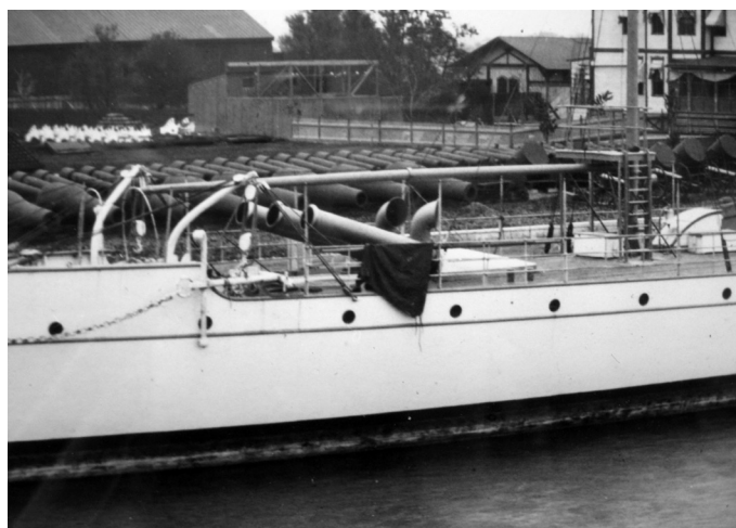
Close up of tubes for pneumatic guns on the USS Vesuvius.
