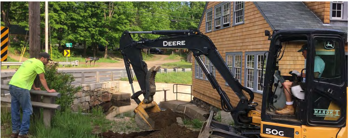
Alec and Jeff Ingram ready to install new signpost
