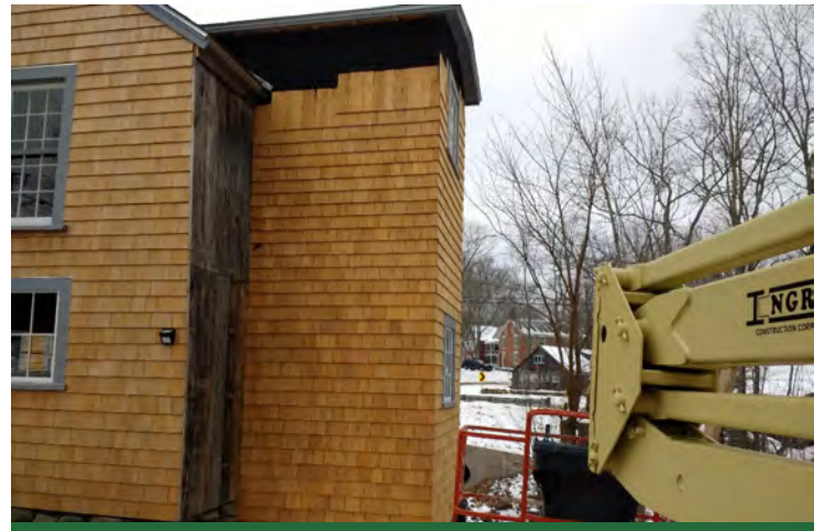
Lift Enclosure Under Construction
