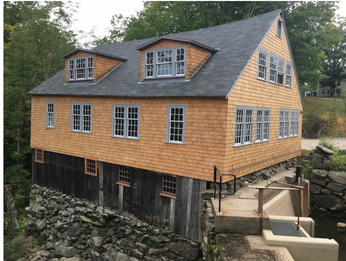
Completed exterior of Chase's Mill, from the northwest
