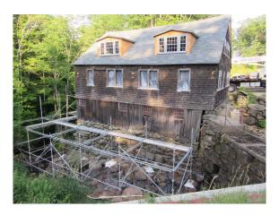
Chase's Mill - early summer 2019 as work is about to begin to restore the windows, replace the siding, and complete repairs to the dam.
